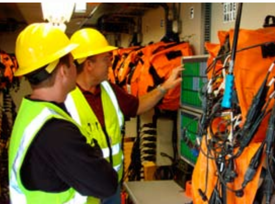
Data is transferred from field units in backpacks via an Ethernet connection while charging batteries.
