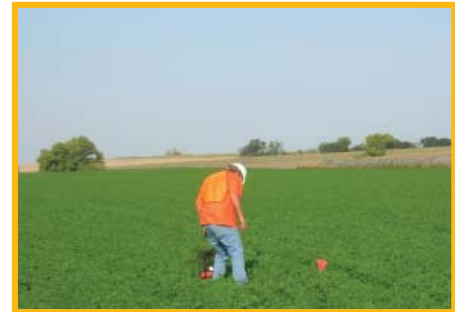
Crew deploying equipment in agriculturally sensitive areas.
